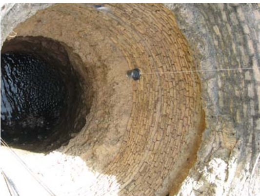
Large diameter dug well
