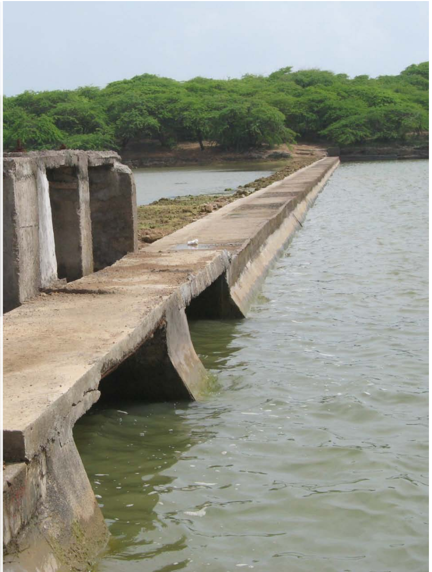
Structure on Kindri creek to control salinity ingress
